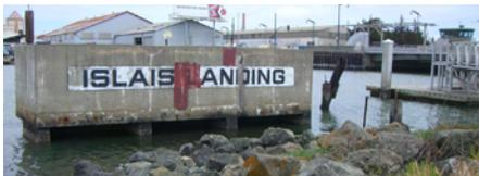
The kayak landing features a floating dock and ramp to accommodate tides. Although it is a new structure, users of the dock would prefer to have it replaced, as the current dock has turns too sharp to negotiate with a kayak.
